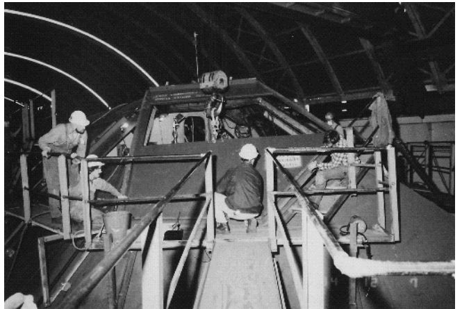
Figure 17. Sea Shadow; Bridge during construction
