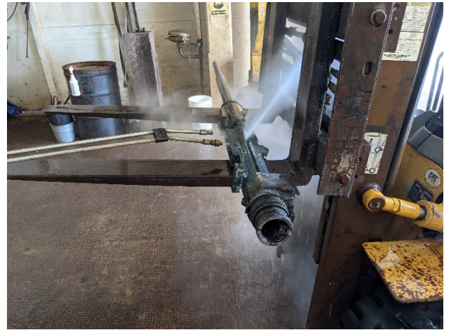
Representative gun being pressure washed to remove loose rust scale and rust chelating agent.
