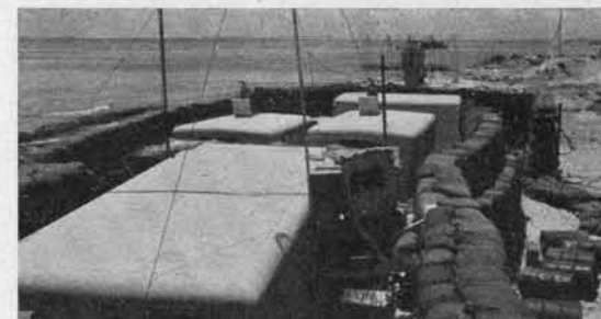
527 operations and power vans revetted. One antenna beyond far end well sited at the water's edge.
